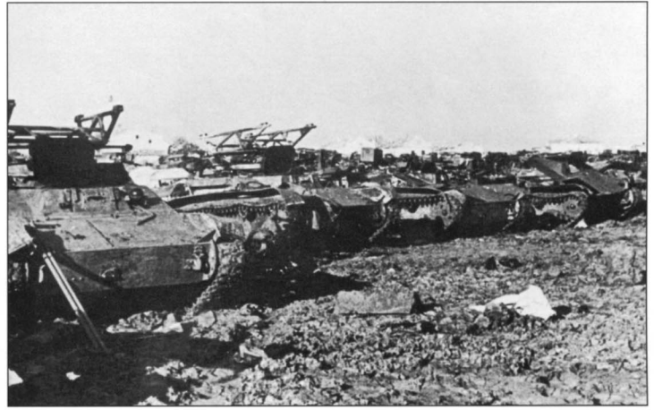
A dumping ground for Soviet armor destroyed in battle and then gathered from the killing fields. All vehicles seen in the first row are T-60 tanks rebuilt into the BM-8-24 vehicle, the so-called "Stalin organ". These "combat machines" (from BM - Boyevaya Mashina) were first produced in the late autumn of 1941 on the T-40 and T-60 chassis following the removal of the turrets and the installation on their mounts of special scaffolding for M-8 missile launchers.
