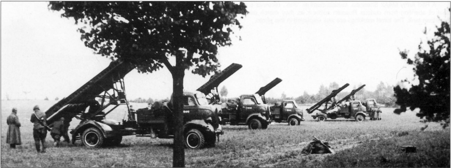
These M-13-16 rocket launchers are each mounted on an American truck, the General Motors COE. Here a battery is ready to fire a salvo. Note the unit markings painted on the cab doors and, particularly, the white circle on the wheels — the Red Army, along with other communist armies, had a special affection for such markings.
