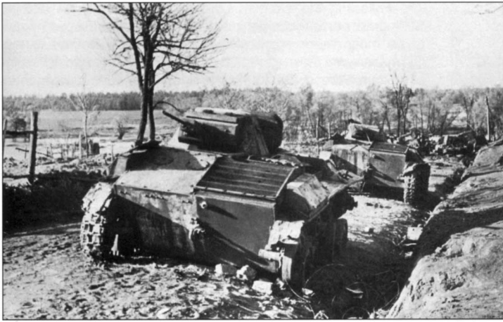
A column of Soviet mechanized troops that were surprised by Germans from the rear and exterminated. In the foreground are two T-60 light tanks with white camouflage. Note that only half of the hull rear plate was painted with white removable paint on both vehicles.
