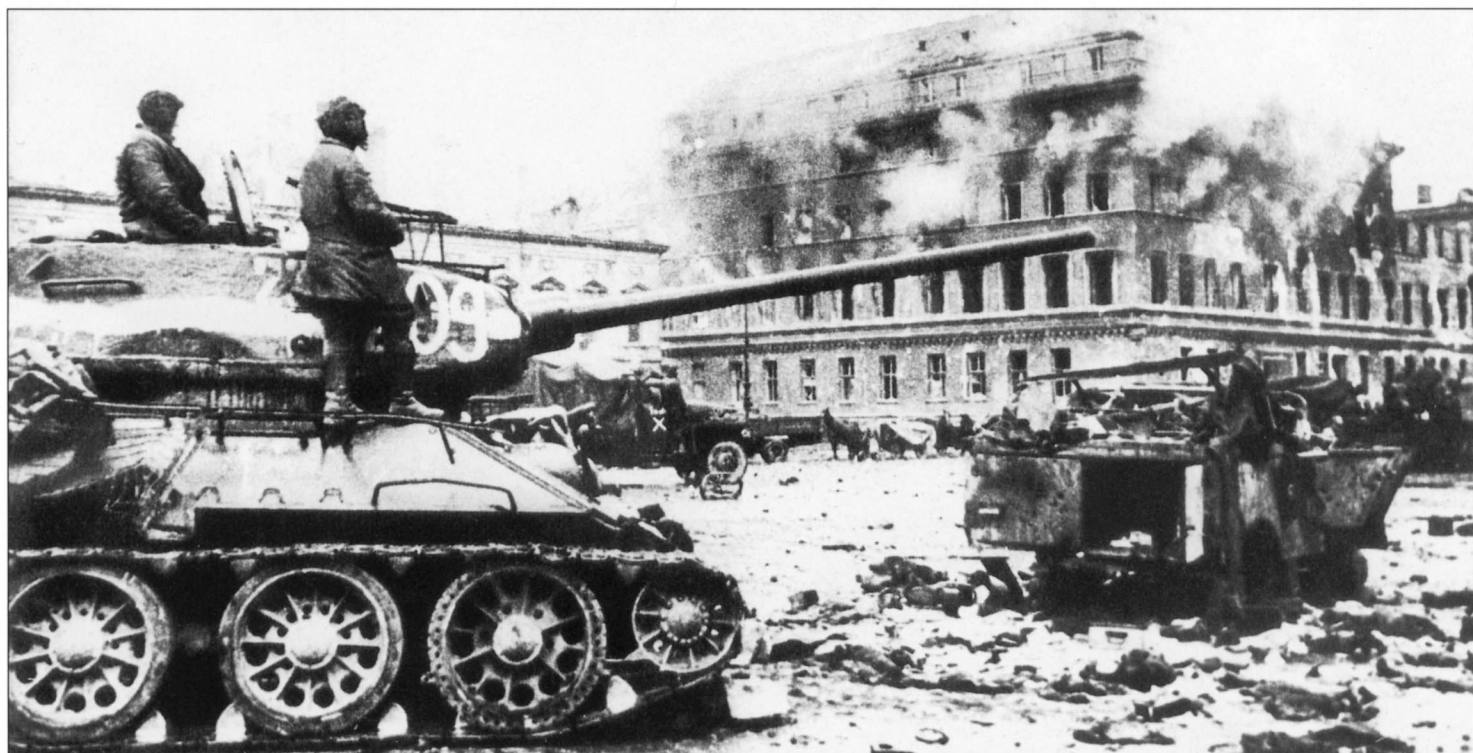
This is a view of the final minutes of the war in the slaughter pen of Berlin. The T-34-85 at the left is marked with a white band around the turret (an Allied recognition sign) and is equipped with wire mesh skirts to protect the tank against Panzerfaust anti-tank weapons. One of them is affixed to the turret in front of the crew hatches. Note that the skirts that were attached to the frontal parts of the turret and superstructure were shot off. Note also the tactical numbers on the turret. One of them is small and painted above the white bar, while another larger one was painted at the same time and with the same paint as the bar. The existence of the unit markings just visible under the number "09" could be explained if the tank carries the markings of two units that used the tank within a few days.
