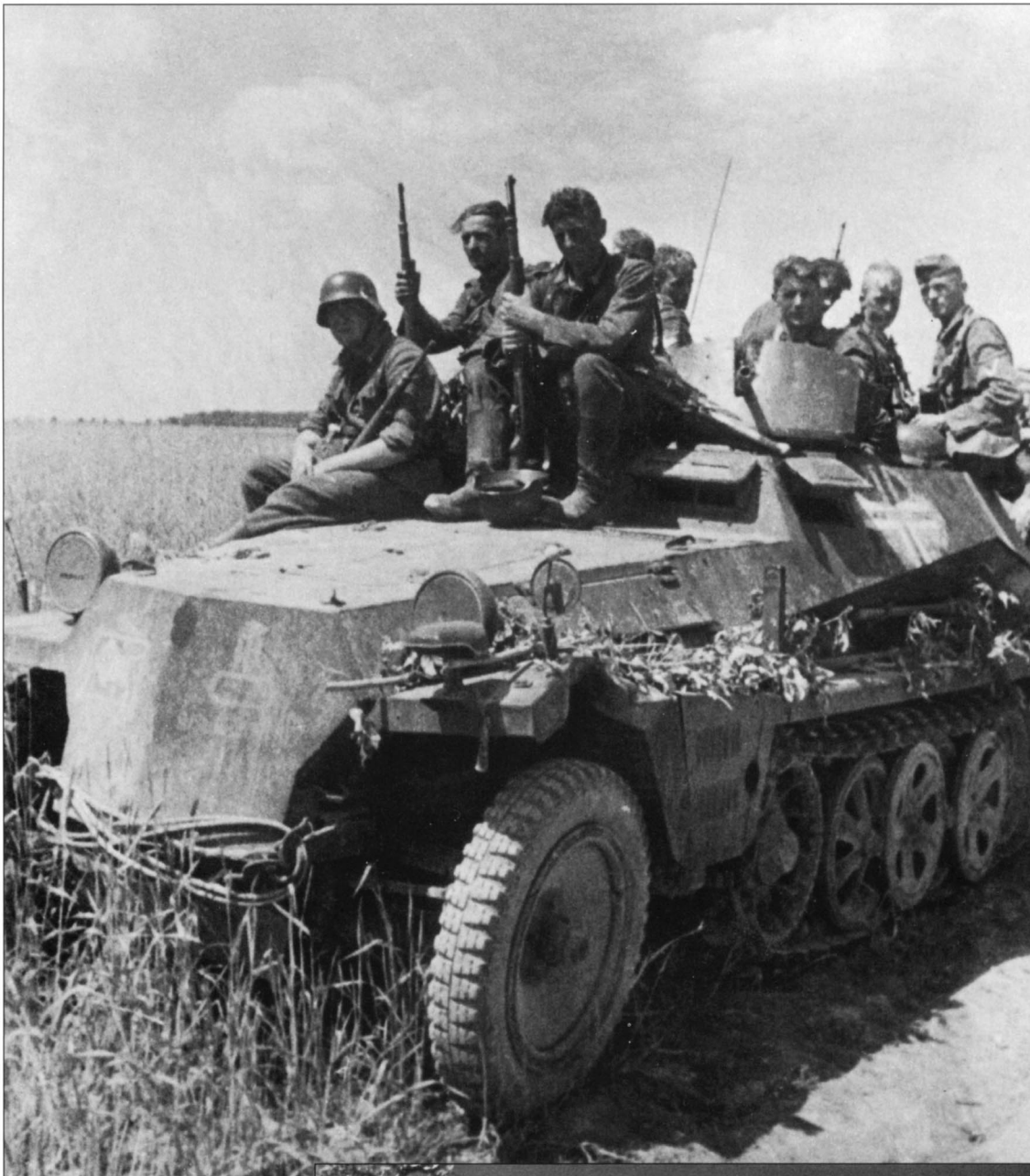
A Sd.Kfz. 250/1 sits at the side of a road loaded down with a squad of stormtroops. This half-track belonged to a StuG battery from StuG.Abt.191, which was employed by Herresgruppe Sud throughout most of 1943, mainly on the Kuban bridgehead. Note that the front plate of the engine armor features a number of markings but lacks a license plate. The unit emblem is visible at left and on the right is the tactical sign.
